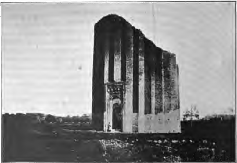
TOWER AMONG THE RUINS OF REI, BEFORE RESTORATION
